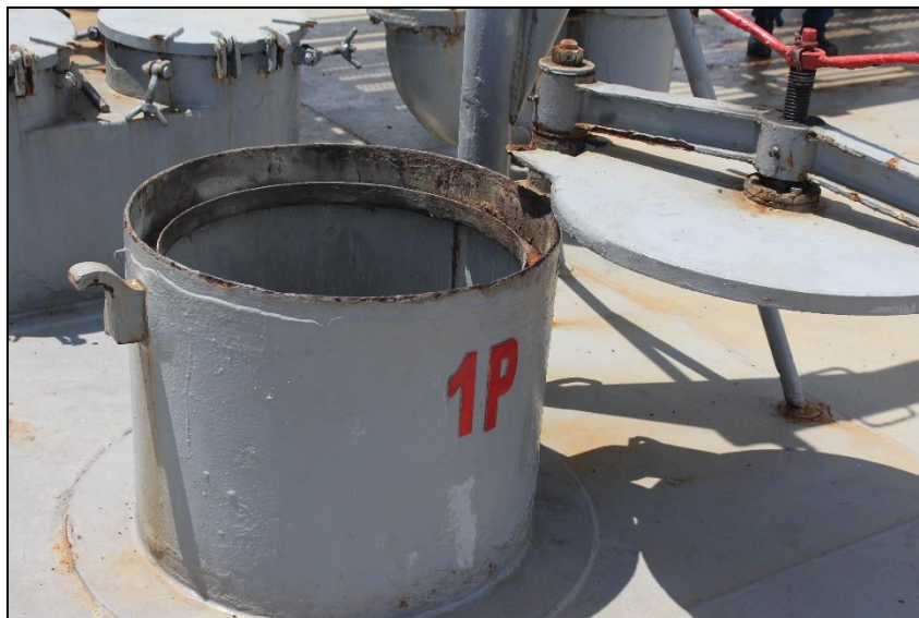
Gambar I-2: hatch cover tipe rotating oil tight Tangki No. 1 Kiri
