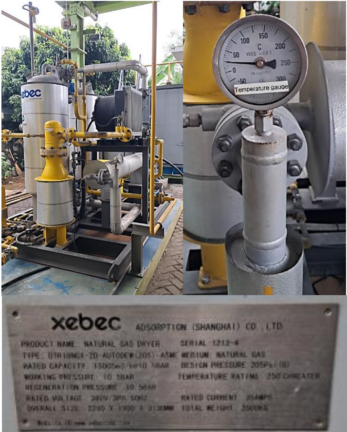
Gambar 25. Air Drier system
